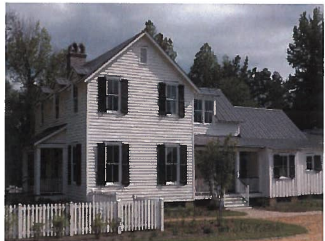
This house design uses ancillary massing (and changes in siding material) to compliment the original massing (two-story main body) in a way that relays an implied story about the history and evolution of the house.
