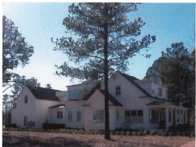
Building massing should be composed of clear forms with secondary masses subordinate to the primary mass.
